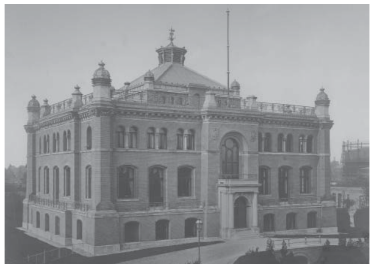
historical view of the building
