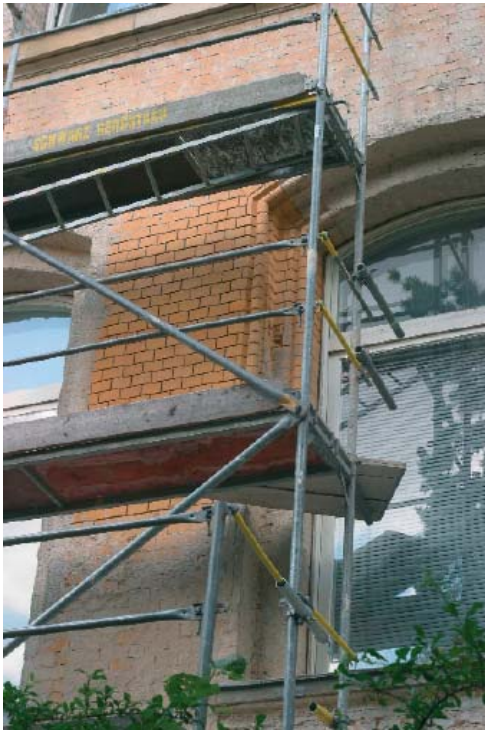
sample area of the restored façade
