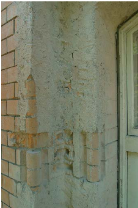
actual condition of the façade
